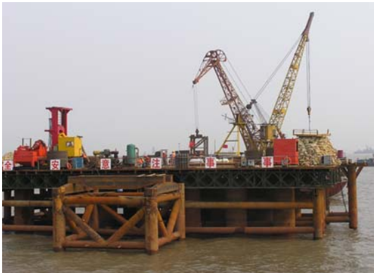
Figure 6: Staging Platform for Piling
