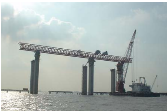
Figure 12: LG Assembling
