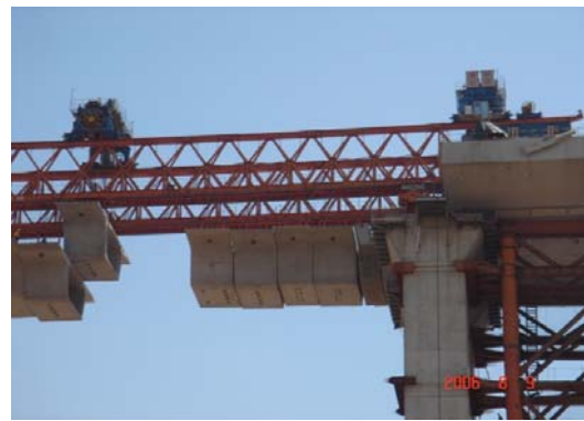
Figure 13: End Span Erection
