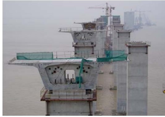
Figure 14: Erected Diaphragm Segment
