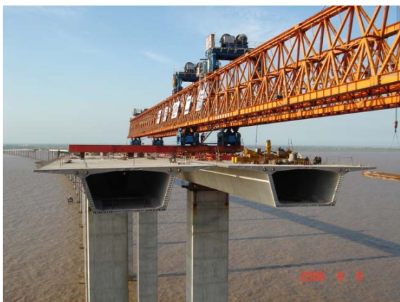
Figure 15a, 15b: Partially Erected Bridge Deck
