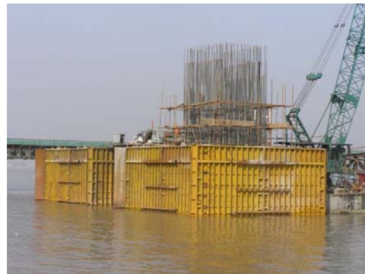
Figure 7: Pilecap Construction
