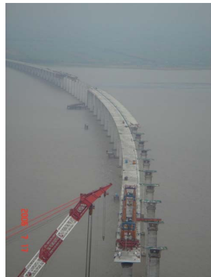
Figure 15a, 15b: Partially Erected Bridge Deck
