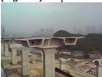
Figure 5 – T-pier with bridge segments stitched
