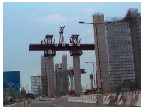
Figure 14 – Plate girder falsework for construction of portal beam
