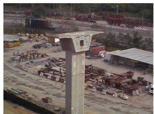
Figure 4 – Precast segment on pier monolithically
