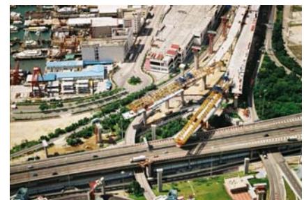
Figure 6 – Erection of segment by launching girder over WKH
