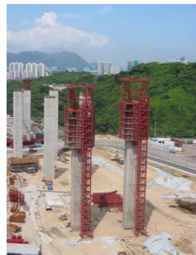
Figure 13 – Self-climbing form for construction of column
