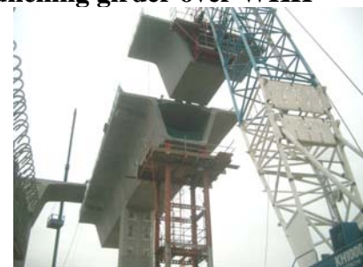
Figure 7 – Erection of segment by crane
